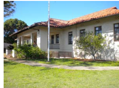
Kaua'i's old courthouse presents an opportunity to revitalize the Līhu'e town core and adaptively reuse a historic building, which is often the approach used by NOAA when considering capital projects. (Source: FPC)
