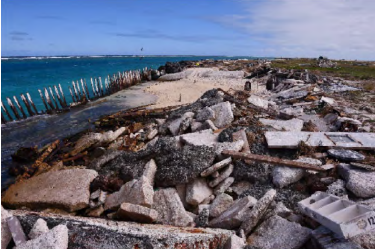
Figure S.PE.4.2. In 2018, Hurricane Walaka removed concrete and sediment covering the Bulky Dump site and exposed potentially hazardous materials. Image: Amanda Boyd/USFWS
