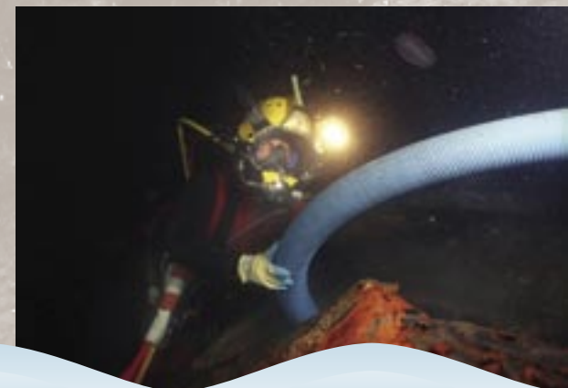
Bobbie Scholley helps remove silt from the USS Monitor 's partially buried steam engine to free it for its salvage lift. Photo: U.S. Navy
