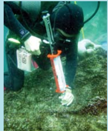
A Galapagos National Park trainee prepares to secure a mooring buoy anchor eye to the bottom. Photo: Amy Massey
