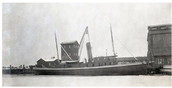
Fig. 21: *Conestoga* being fitted out at the Maryland Steel Company's Marine Department shipyard. The photograph was probably taken soon after its launching since the tug's name is visible on the name board, but has not been added to the bow, a requirement of United States Bureau of Navigation.
