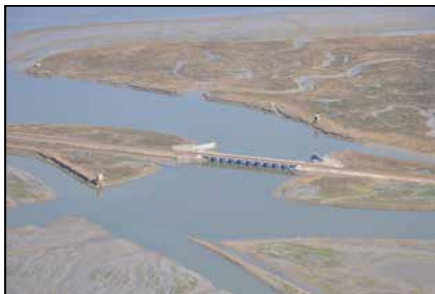
Figure 6. Aerial photo of a sill that was installed at the mouth of Parson’s Slough in 2011. The purpose of this restoration project was to reduce erosion and wetland loss in Elkhorn Slough.
