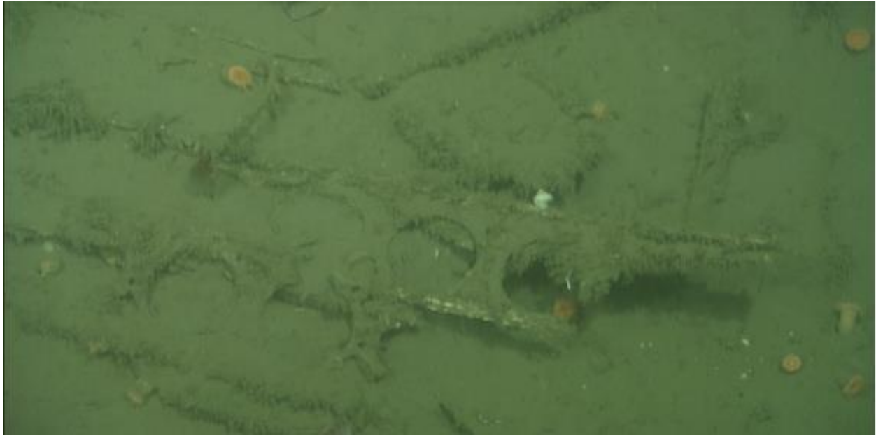
Figure 10- Disarticulated box girder, Field A (NOAA, MBARI 2007)
